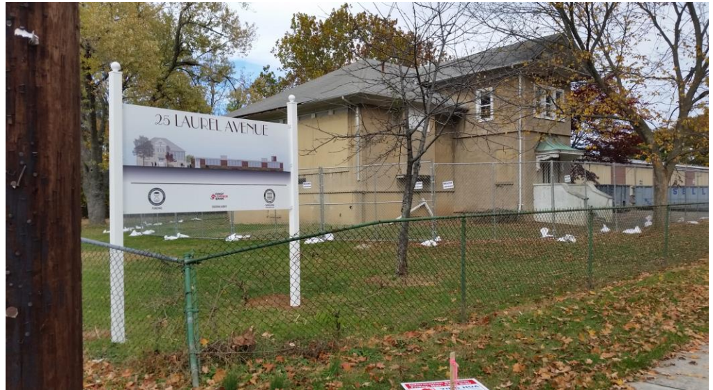
25 Laurel Ave has been unoccupied with boarded windows for over 10 years. Construction began in October.
